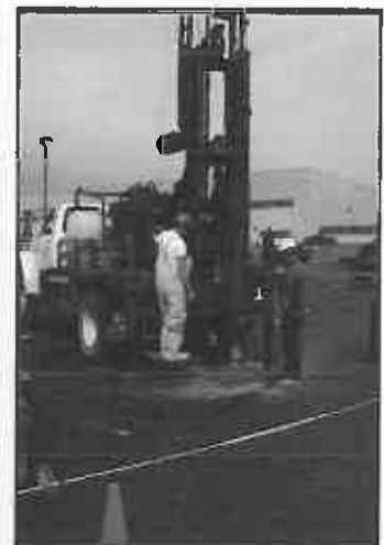
Drilling on Flat Terrain
