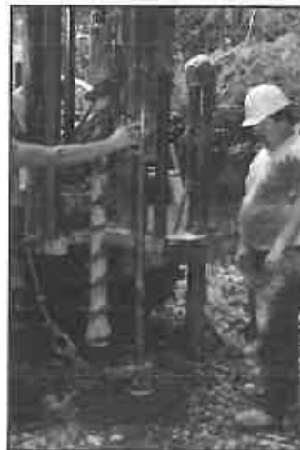
Drilling in Rough Terrain
