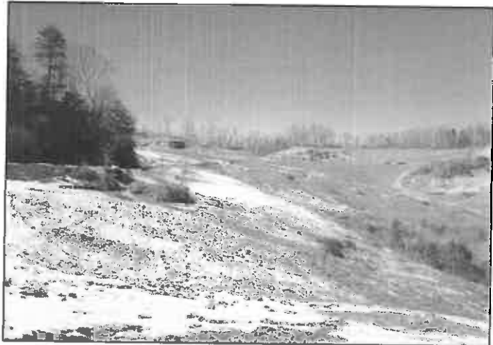
Portions of the landfill were steeply sloped which presented a challenge in designing the geosynthetic cap system.
