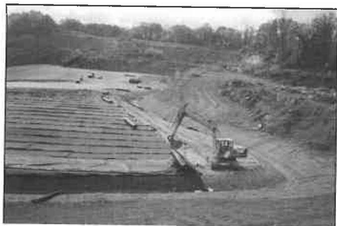
The project included construction of a 19-acre geosynthetic cap system.
