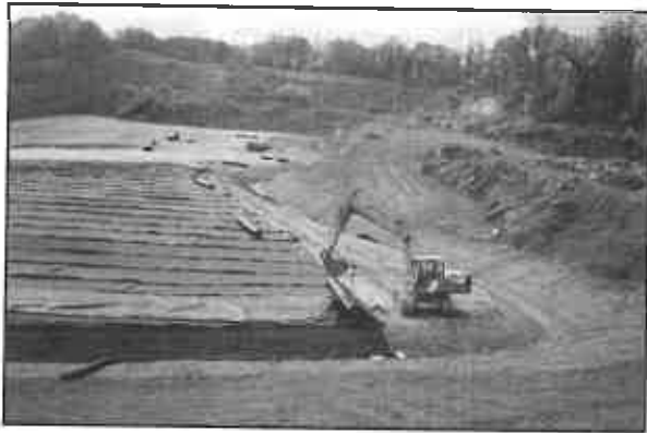
The project included construction of 19 acres of a geosynthetic cap system.
