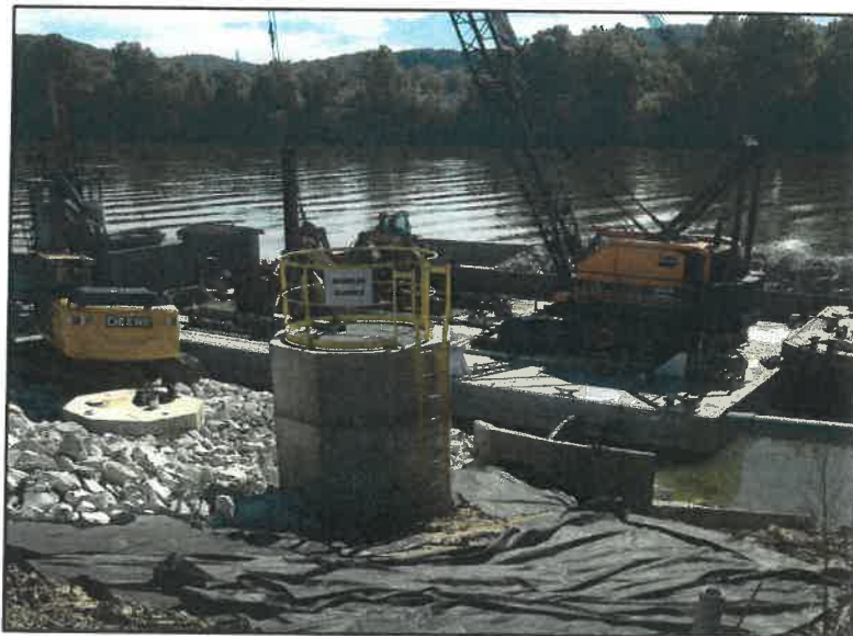
Degassing Overflow Manhole during Construction, with Kanawha River in Background
