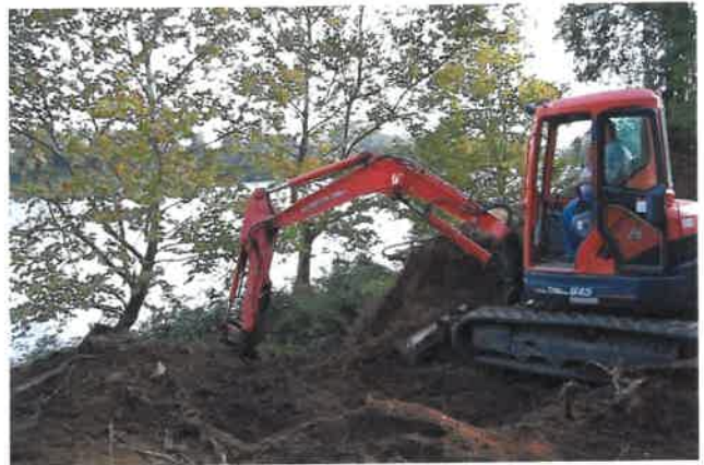
Monitoring of excavator creating trench to accommodate new boat docking facility.
