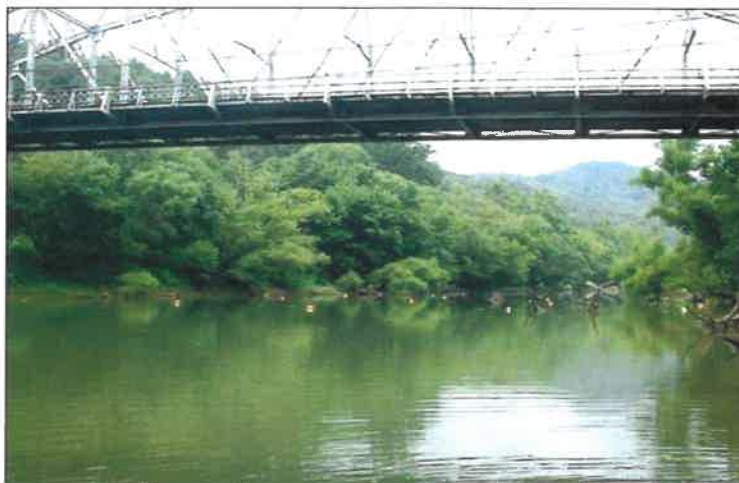
The Old Lower Gassaway Bridge over the Elk River, Orange Buoys Demarcate Mussel Survey Search Cells.
