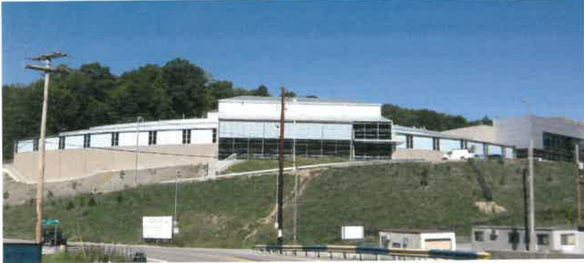
HVAC at LEED Certified Hilltop Elementary School
