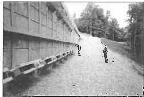
Finished wall with anchors
