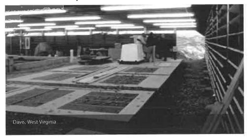
E.L. Robinson Engineering Co. was contracted by the West Virginia Division of Natural Resources, Parks & Recreation to design a new concrete sewage treatment plant which eliminates the potential for rust. The new plant also uses ultraviolet disinfection and provides a sand filter prior to discharge into the Blackwater Canyon.
