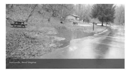
ELR prepared construction documents for mitigating the standing water present in many of the 26 sites due to years of added road pavement and lack of adequate cross slope and drainage swales throughout the campground.
