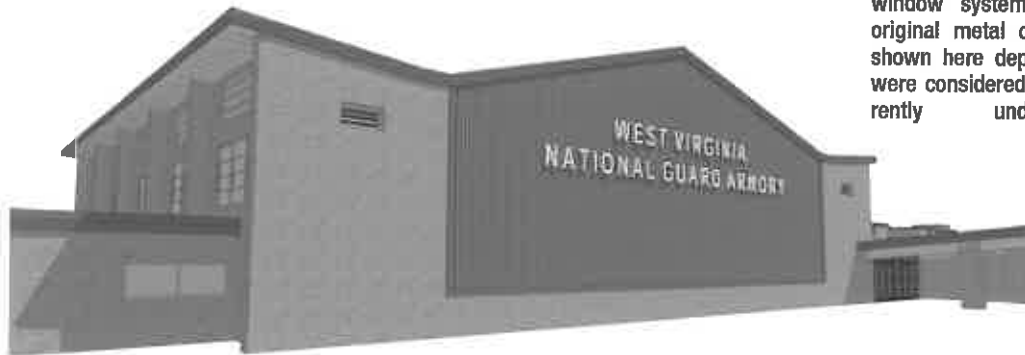
Existing Metal Facade
