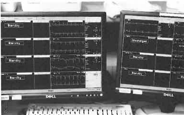
Alarm details are available at the central station and on the mobile device.
