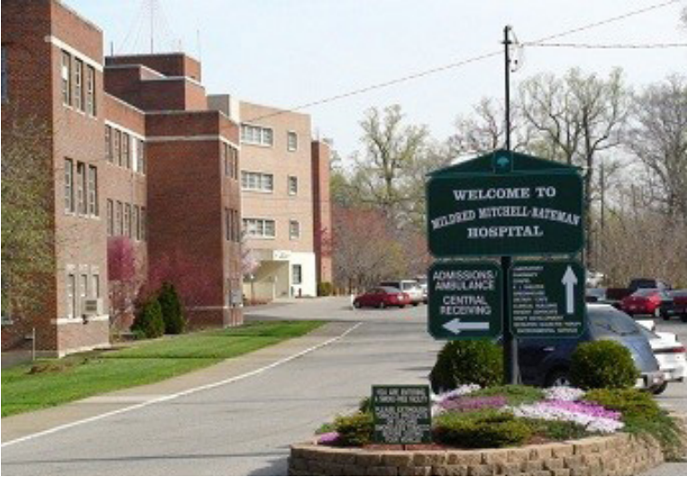
MILDRED MITCHELL-BATEMAN HOSPITAL Huntington, WV
