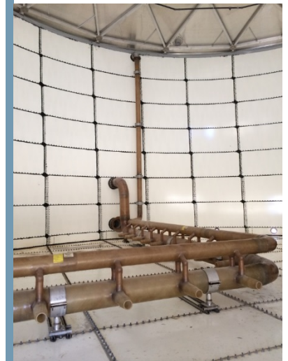
Inside of newly constructed tank
