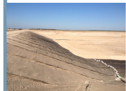
Cell Construction – March 2013
