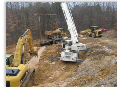
*Installation of biopolymer slurry
