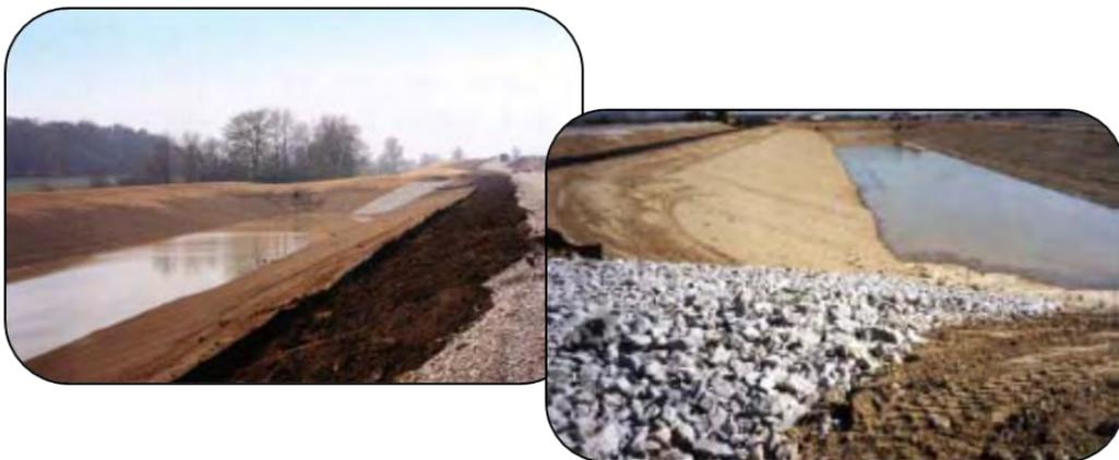
B&N was retained by the Solid Waste Authority of Central Ohio to provide plans and specifications for Sediment Pond No. 1 and a new access road embankment. The sediment pond and access road were needed as a part of the future expansion of the landfill. Construction plans and specifications were developed from Permit-to-Install drawings for the landfill expansion.
