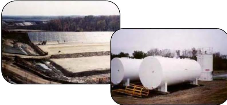
B&N was retained by WCI Steel, Inc. to provide detailed design services for the construction of a new leachate transfer system for its Warren, Ohio plant. WCI Steel operates a residual solid waste disposal facility for on-site disposal of residual wastes generated through the steel making process. Liquid that accumulates in the solid waste disposal facility is considered landfill leachate and is required to be handled in accordance with Ohio EPA regulations.
