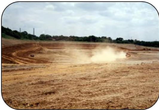
B&N was retained by the Cincinnati Gas & Electric Company to prepare construction plans for a newly permitted landfill to receive ash from the Miami Fort Power Station. This new landfill incorporates a multiplayer bottom liner system consisting of a recompacted clay liner beneath a geomembrane and leachate collection system.
