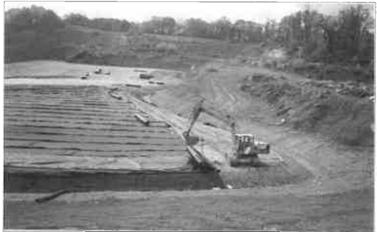
The project included construction of 19 acres of a geosynthetic cap system.
