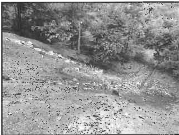
Exposed Refuse Pile with Erosion
