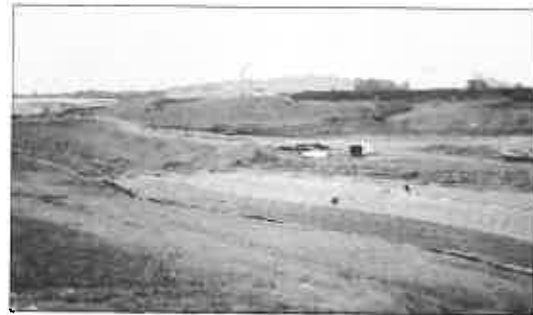
Construction of the HDPE geomembrane over Cell F-3b.
