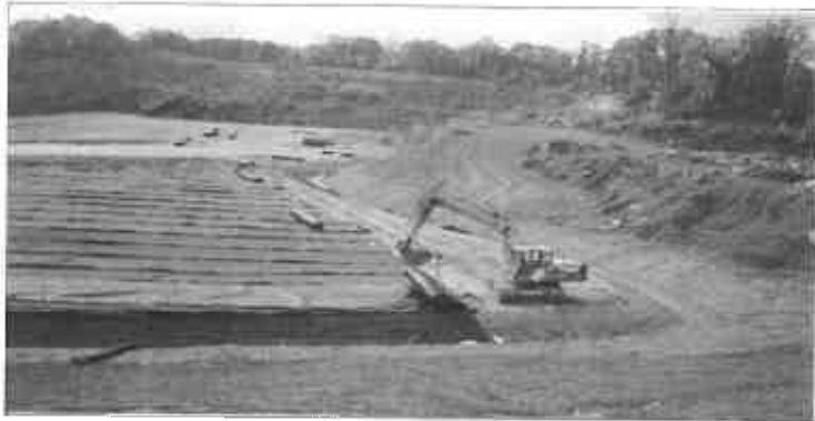
The project included construction of a 19-acre geosynthetic cap system.
