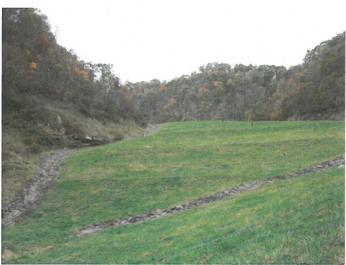
The closure cap consisted of 18 inches of intermediate cover soil material, geocomposite gas venting and leachate collection layers, 40 mil linear low density polyethylene (LLDPE) flexible membrane liner, and a 24 inch vegetative soil cover layer.
