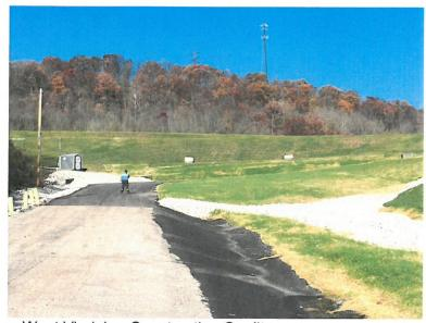
Engineering, Inc. (Triad) of St. Albans, West Virginia. Construction Quality Assurance/Quality Control monitoring and materials evaluation were also performed by Triad. The repairs consisted of collecting and properly sealing seeping waste and leachate and repairing the access road.
