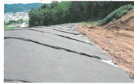
Triad Engineering, Inc. (Triad) of St. Albans, West Virginia. Construction Quality Assurance/Quality Control monitoring and materials evaluation were also performed by Triad. The construction of the Phase I Expansion consisted of installing a liner in the unlined portions of the western side of the landfill and closure of an interim capped area.
