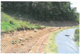
also being performed by Triad. The construction of the Expansion is currently ongoing and consists of raising the crest of the existing earthen dam and adding berms and walls.
