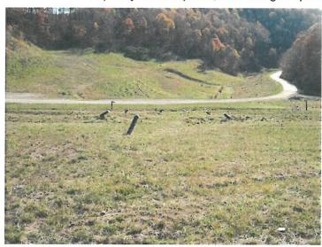
The intent of the proposed closure plan systems was to; minimize surface water infiltration, thereby minimizing generation of leachate, collect and remove any surface and/or subsurface leachate seepage, collect and remove gas generated during waste decomposition, and to minimize the potential for erosion of the closure cap by surface water run on/runoff.
