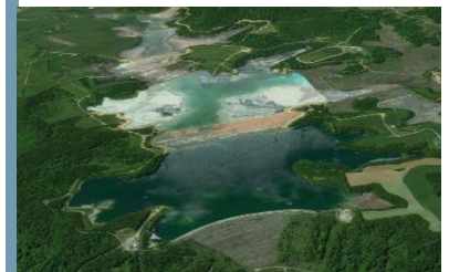
The 965-acre CCR disposal impoundment is contained behind a rock-fill dam measuring 2,200 feet wide at the crest and 400 feet tall.
