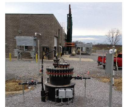
Condensate sump of gas collection and control system
