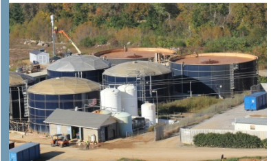
Leachate Pretreatment Facility
