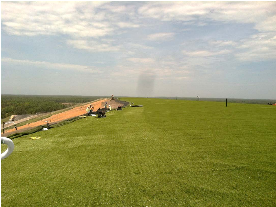
Installation of the ClosureTurf Final Cover System on the top deck.
