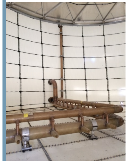
Inside of newly constructed tank
