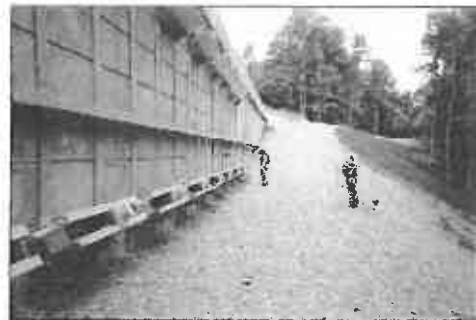
Finished wall with anchors
