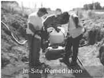
Underground Storage Tank Removal
