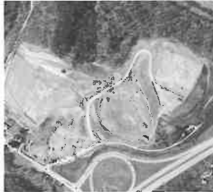
Gateway Development Site: I-79 Exit 155
