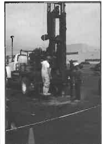
Drilling on Flat Terrain
