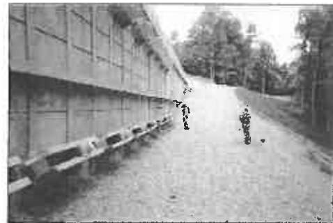
Finished wall with anchors
