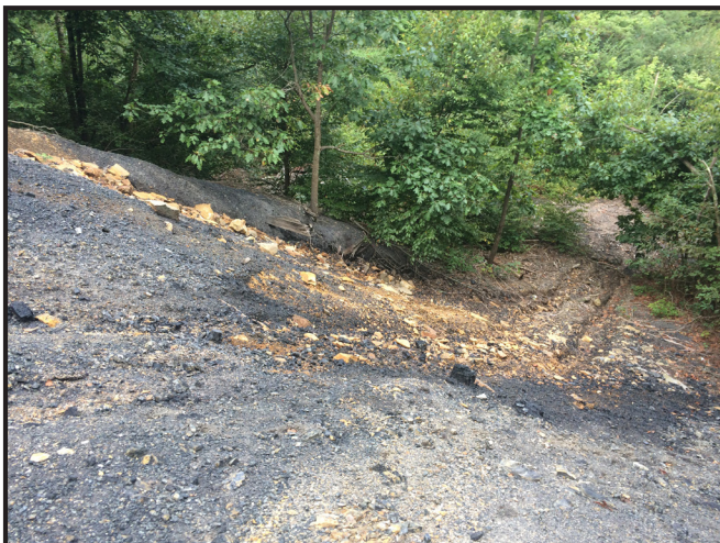
Exposed Refuse Pile with Erosion
