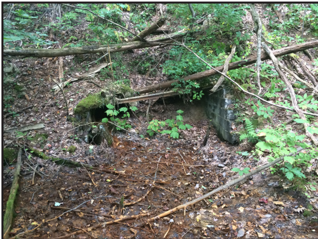
Collapsed Portal Structure
