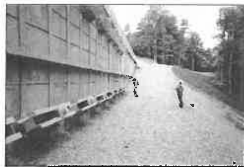
Finished wall with anchors
