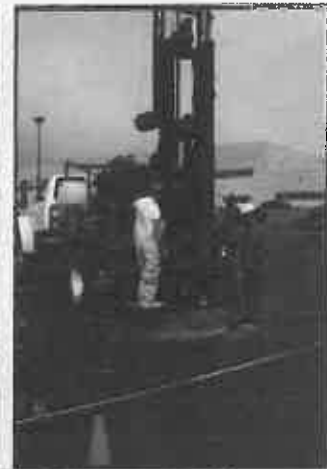
Drilling on Flat Terrain
