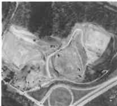
Gateway Development Site: I-79 Exit 155
