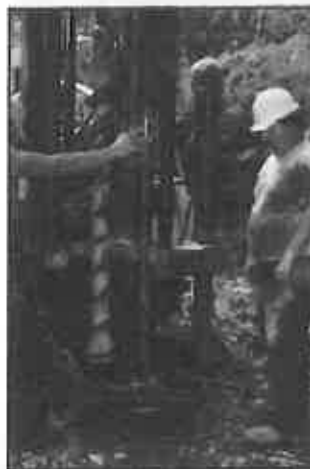
Drilling in Rough Terrain
