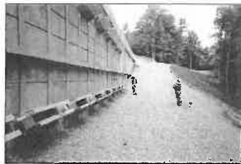
Finished wall with anchors
