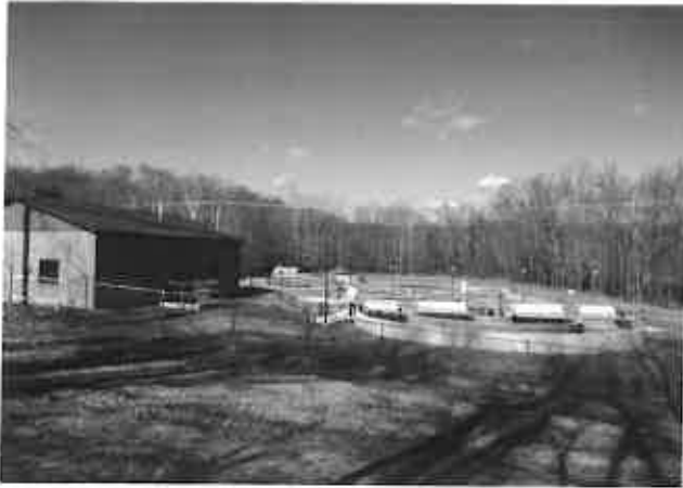
New 0.370 MGD WWTP
