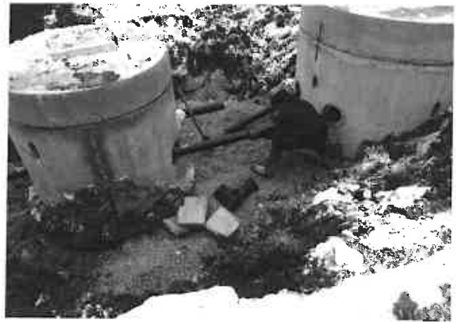
Lift Station Improvements
