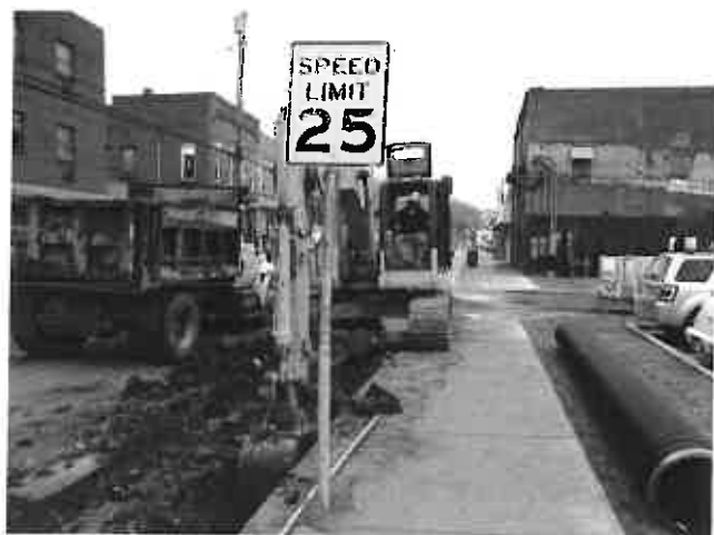
Storm Water Separation on US Route 250
