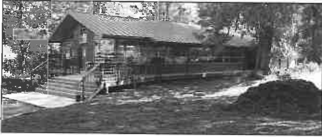
The refurbishment of Camp Fircom featured not only a new AdvanTex wastewater system, but also a dining hall designed by Principle Architecture. Photo courtesy of Camp Fircom.
