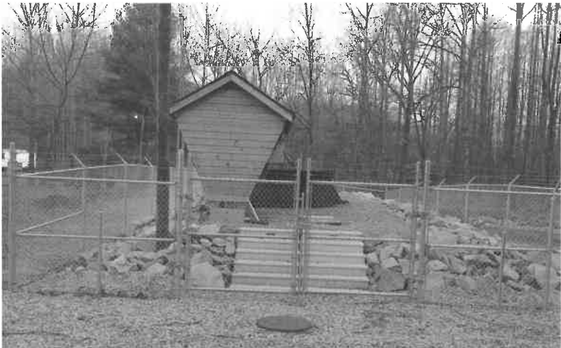
Community of Ury Wastewater Treatment Facility (part of Crab Orchard-MacArthur PSD)
