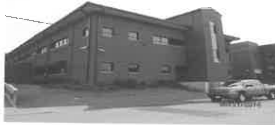
WVDOH-District 1 Administrative Office
