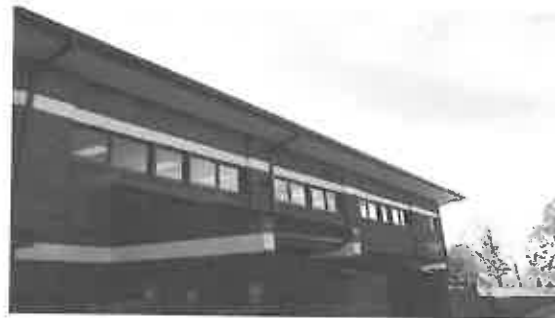
WVDOH-District 9 Administrative Office
