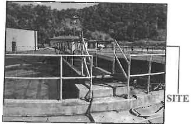
Addition of Third Clarifier
