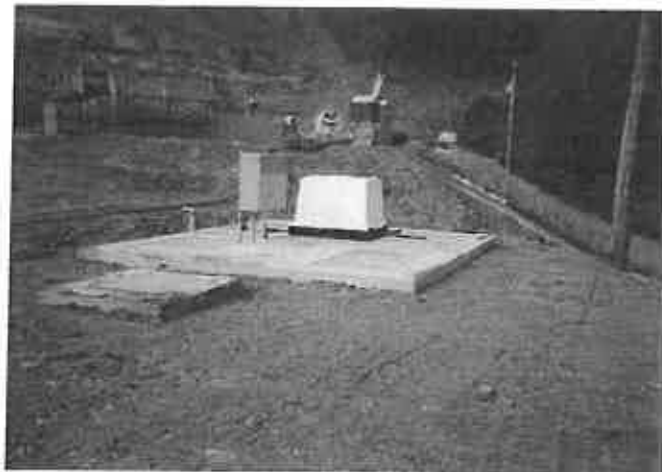
Equalization Tank/Pump Station During Construction
