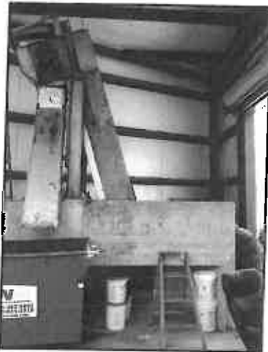
Mechanical Bar Screen to be Replaced
