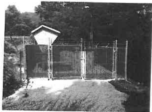
After: Upper Drive Lift Station
