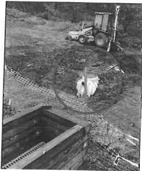
New Chlorine Contact Basin, Under Construction
