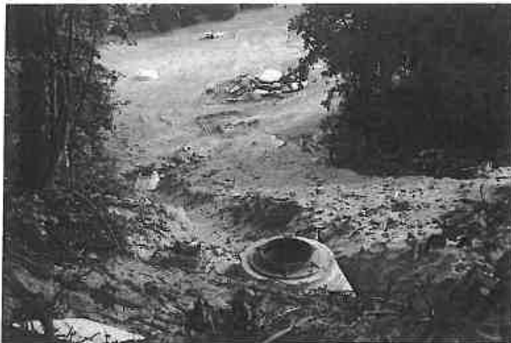
Manhole During Construction
