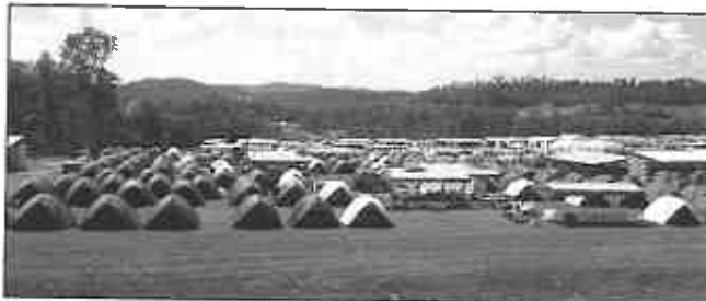
Over 100 AdvanTex AX-RTs at the BSA's national "Jamboree" site treat greywater from sinks and showers for reuse in toilets. Photo courtesy of Tim Felbinger.
