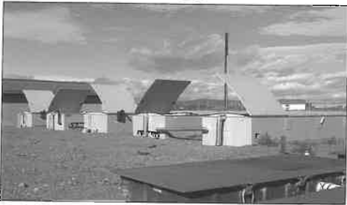
The Yakama Nations Housing Authority in Washington state added five AdvanTex ® AX-Max units (background) to its ten AdvanTex AX-100 units, increasing the capacity of its wastewater system by 50%. Photo courtesy of Fextex Systems, Inc.
