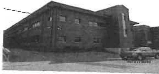
WVDOH-District 1 Administrative Office
