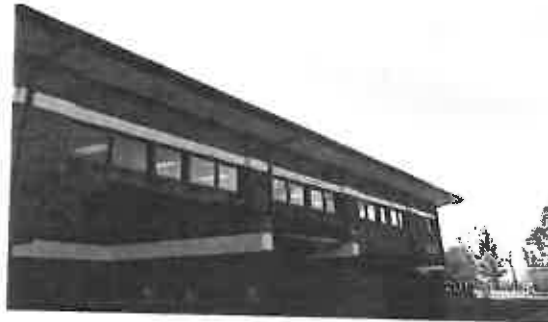
WVDOH-District 9 Administrative Office
