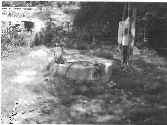
Before: Upper Drive Lift Station
