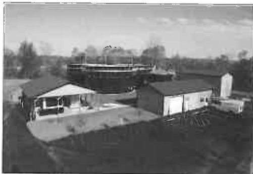
Wastewater treatment plant
