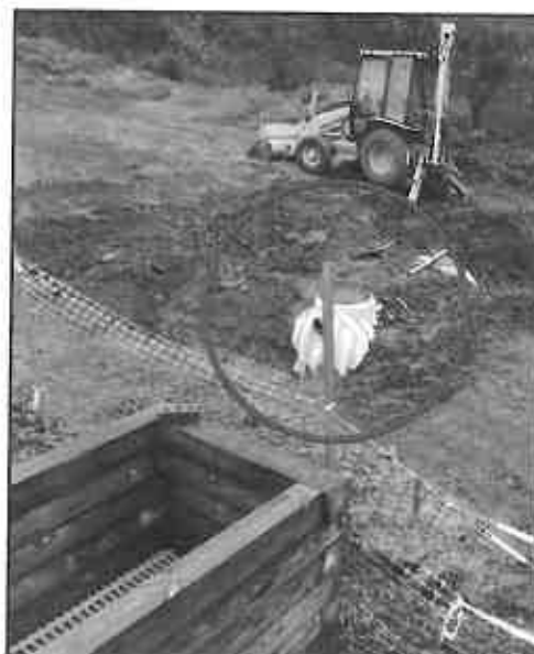
New Chlorine Contact Basin, Under Construction
