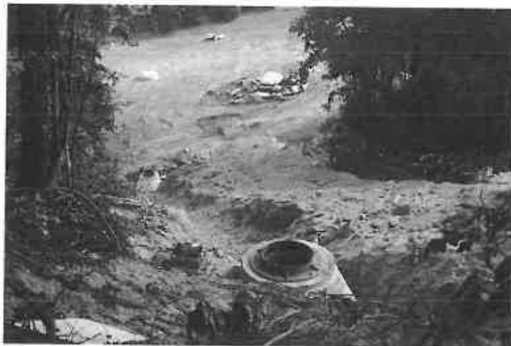
Manhole During Construction
