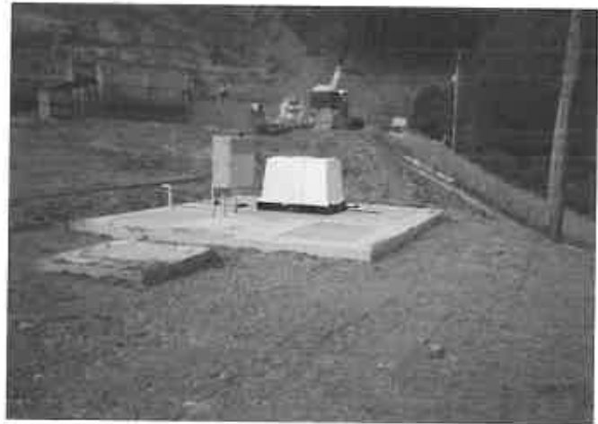
Equalization Tank/Pump Station During Construction
