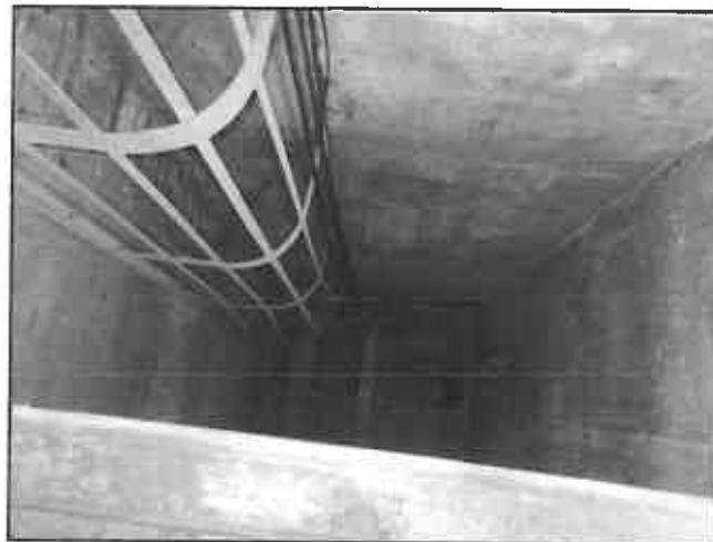
Wet Well of Pump Station to be Rehabilitated
