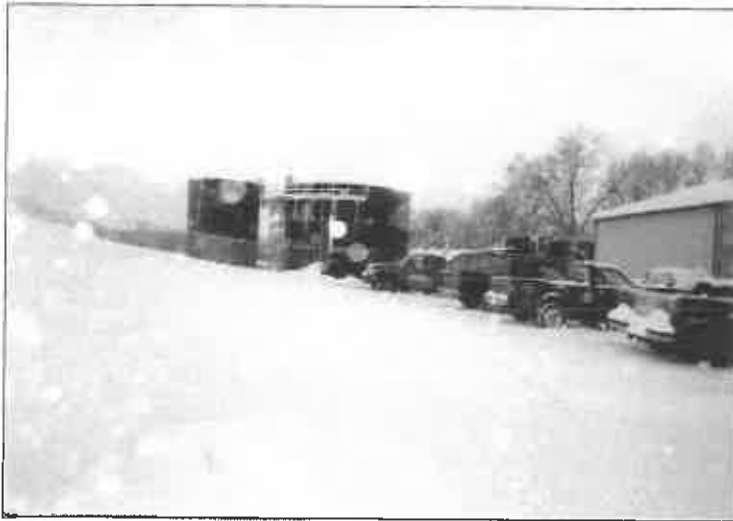
Aerobic digester tank (left) and SBR tank (right)
