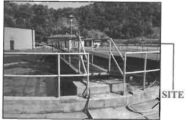
Addition of Third Clarifier
