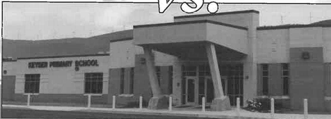
Completed School in 2013
