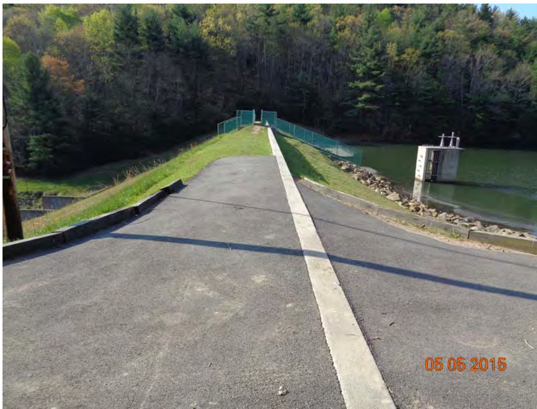
LONG BRANCH DAM MODIFICATION, PIPESTEAM STATE PARK
