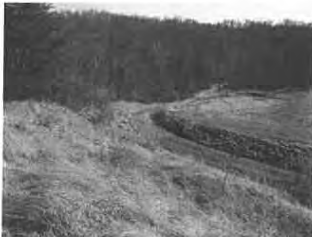
Photo No. 3: Emergency spillway outlet.
