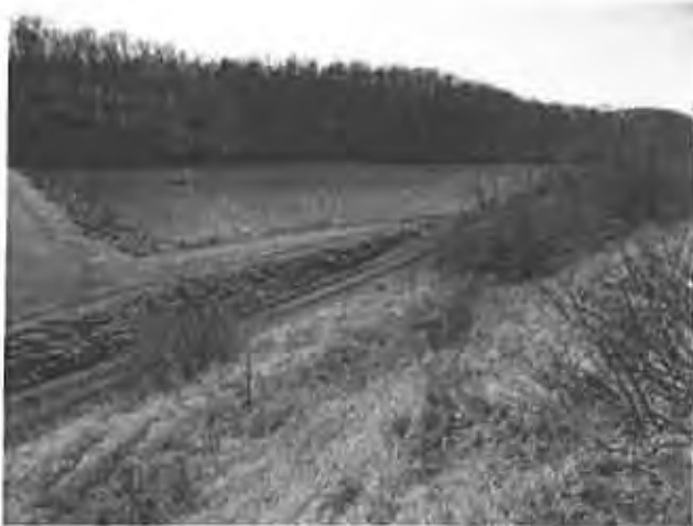
Photo No. 2: Emergency spillway entrance.
