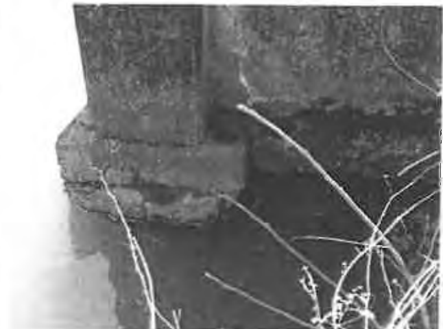
Photo No. 23: Close-up of erosion and undermining.
