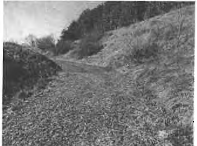
Photo No. 5: ESW facing upstream.
