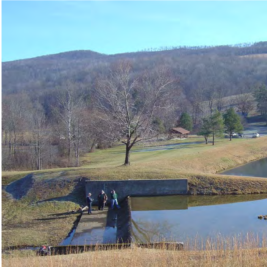
BELINGTON DAM MODIFICATION, BELINGTON, WV
