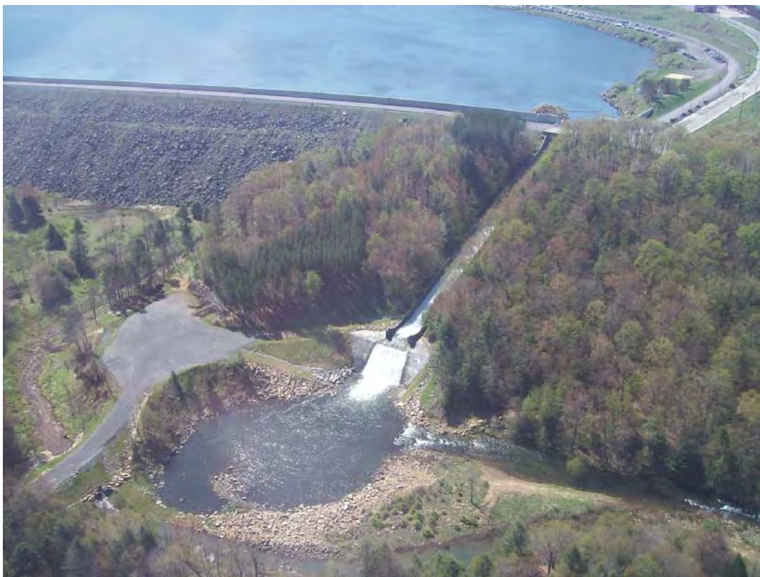
MT. STORM FLIP BUCKET STABILIZATION (RCC), MT. STORM POWER STATION
