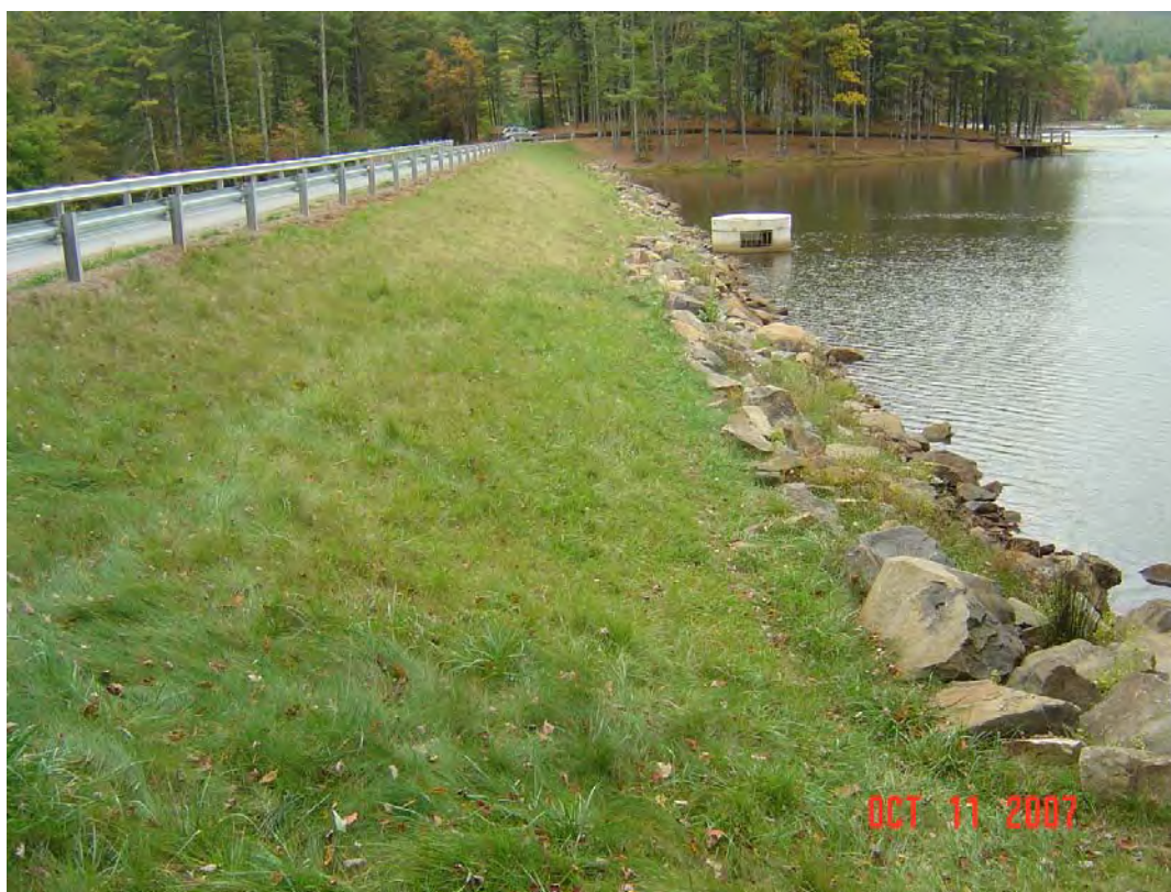
MONCOVE DAM MODIFICATION, MONROE CO., WV
