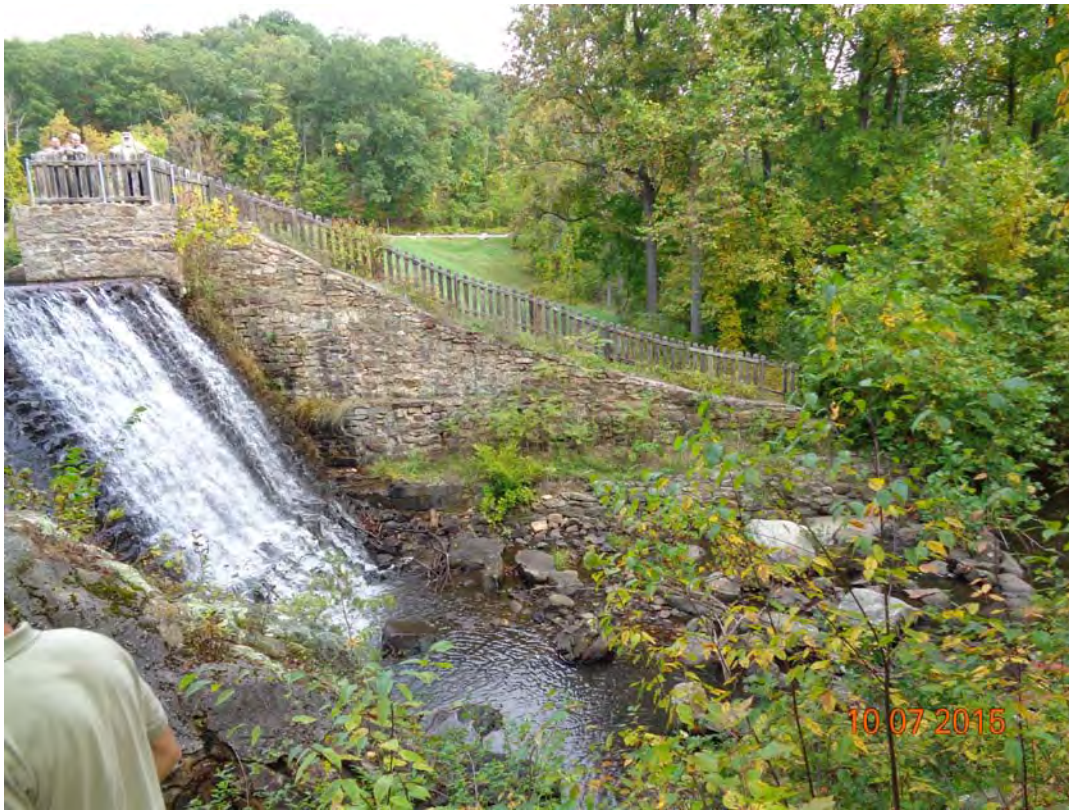
PARK DAM MODIFICATION (RCC), CACAPON STATE PARK
