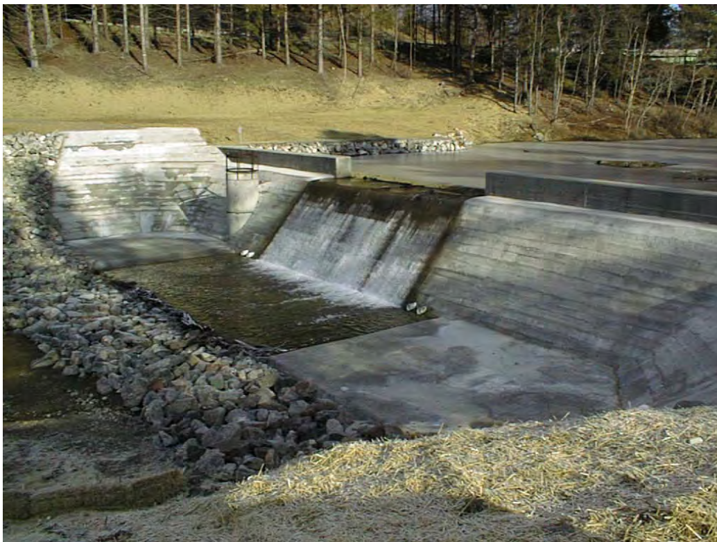
THOMAS DAM MODIFICATION, THOMAS, WV
