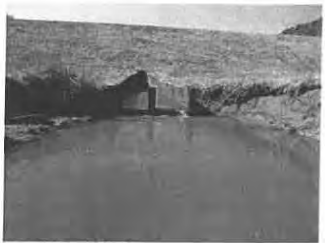
Photo No. 16: PSW outlet structure and plunge pool.
