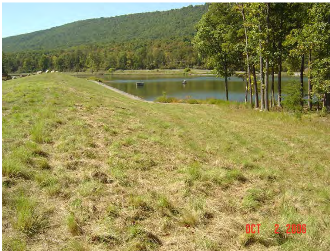
WARDEN LAKE DAM MODIFICATION, HARDY CO., WV
