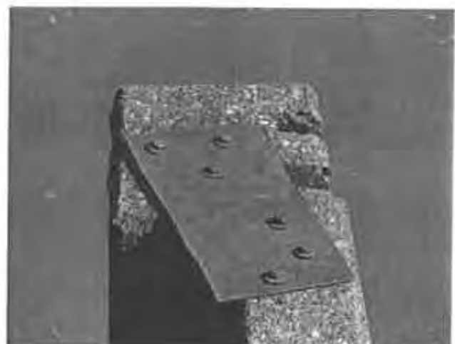
Photo No. 24: Steel plate repair.
