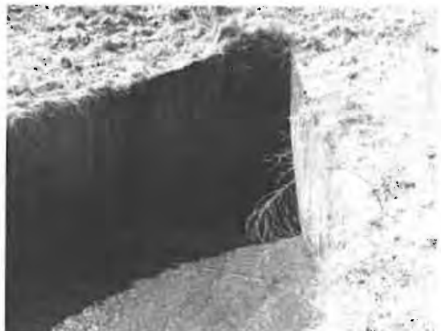
Photo No. 18: Pipe outlet.
