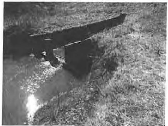
Photo No. 22: Erosion adjacent to the outlet structure.
