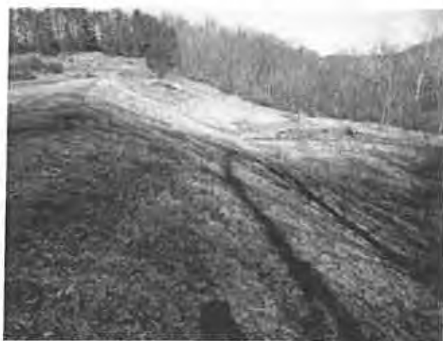
Photo No. 10: Downstream slope facing left.
