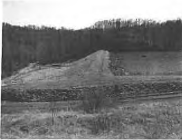
Photo No. 1: Overall view of dam.
