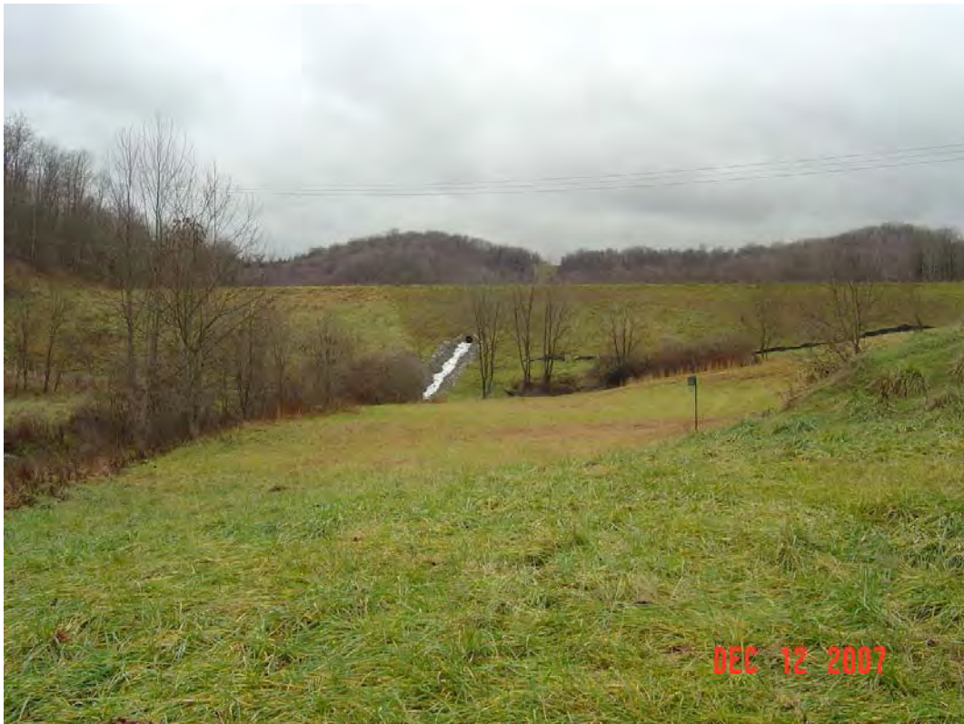
LEMLEY DAM MODIFICATION, MONONGALIA CO., WV
