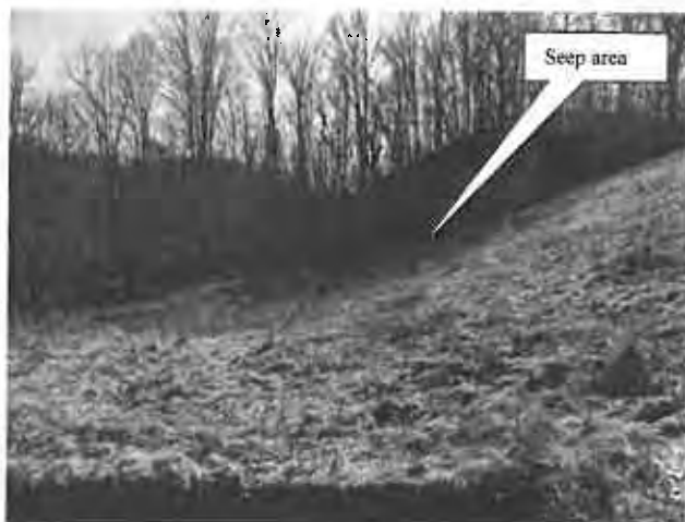
Photo No. 12: Right groin.
