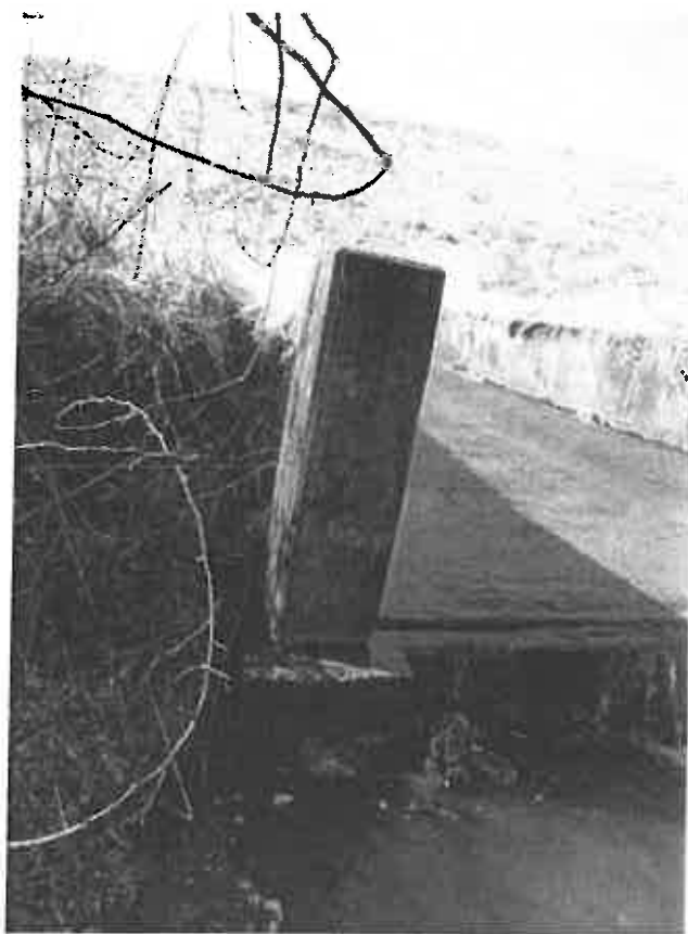
Photo No. 25: Right wall tilt.
