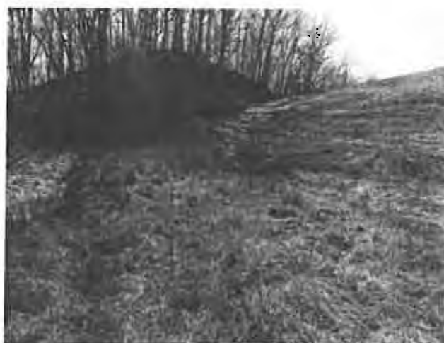
Photo No. 11: Right groin and seep area.
