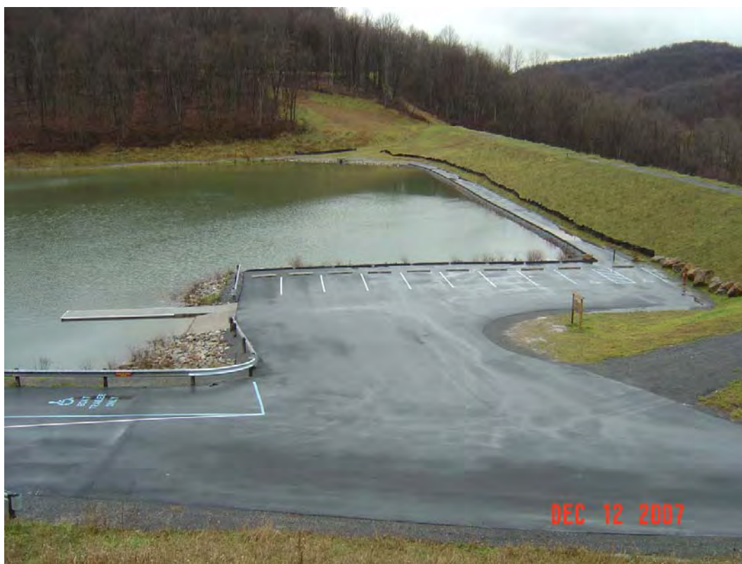
BAILEY DAM MODIFICATION, MONONGALIA CO., WV
