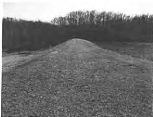
Photo No. 8: Dam crest facing right.
