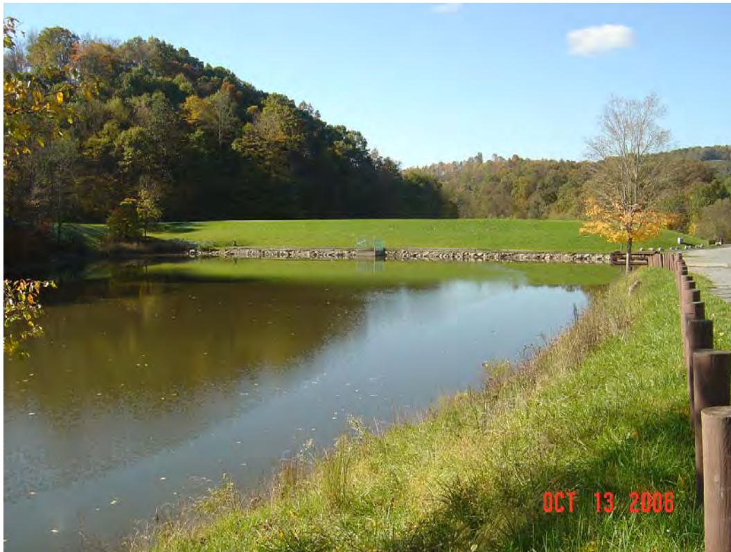
JIMMY LEWIS DAM MODIFICATION, MERCER CO., WV
