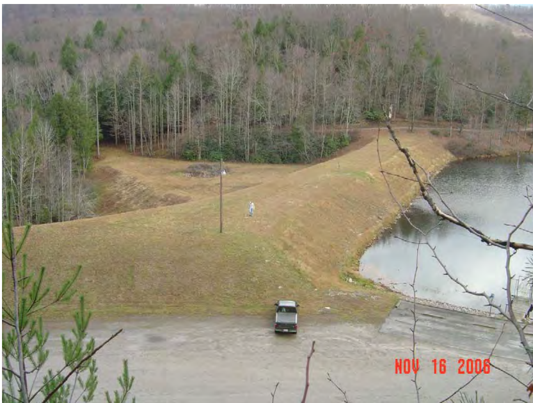
PLUM ORCHARD DAM MODIFICATION, FAYETTE CO., WV
