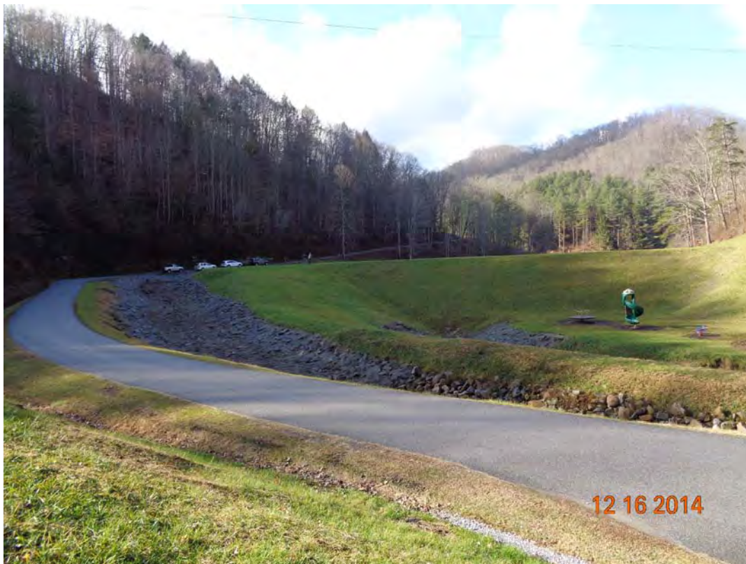
BERWIND DAM MODIFICATION (RCC), MCDOWELL COUNTY, WV
