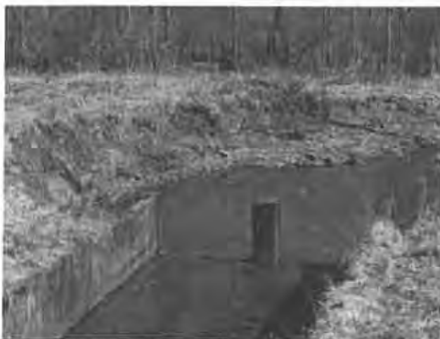
Photo No. 21: Erosion in plunge pool at end of outlet structure.
