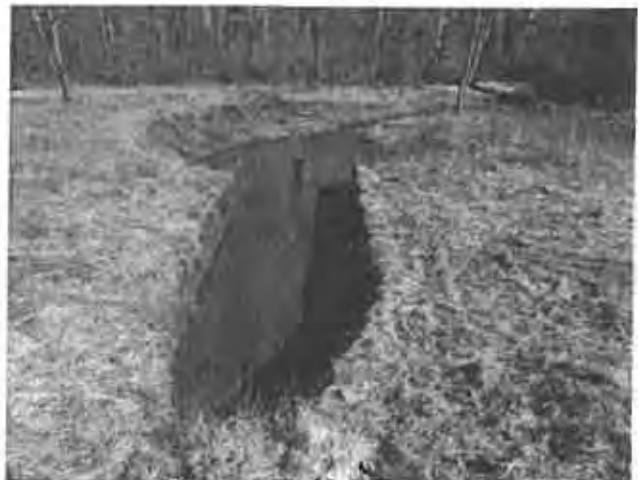
Photo No. 17: PSW outlet structure and plunge pool.
