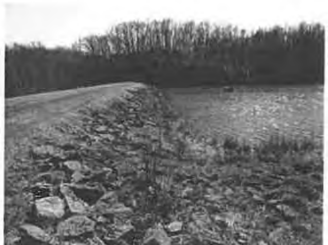
Photo No. 6: Upstream slope facing right.
