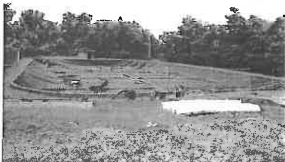
Reservoir Floating Cover Replacement
