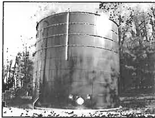
402,000-Gallon Water Storage Tank
