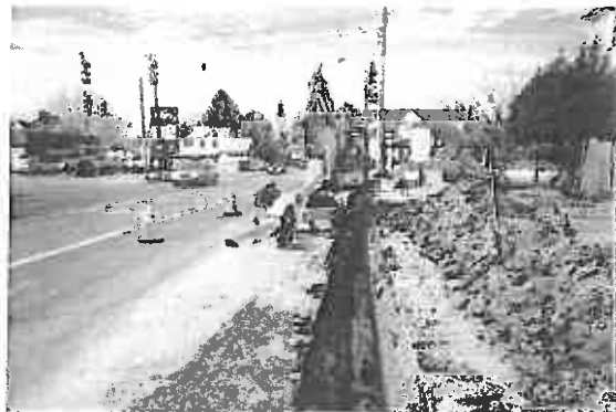
Replacement of water line along US Route 60.
