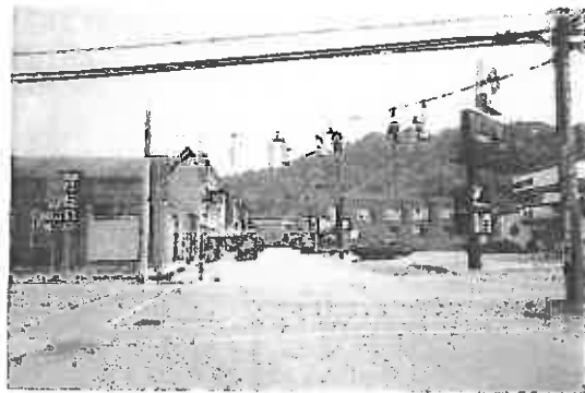
Main Street Where 8" Water Line Was Installed
