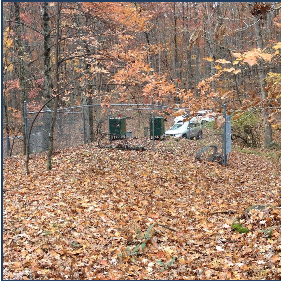
Picture 1 Babcock State Park WWTP
