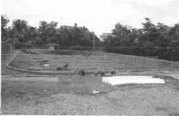
Reservoir Floating Cover Replacement
