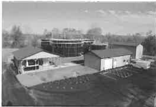
Wastewater treatment plant
