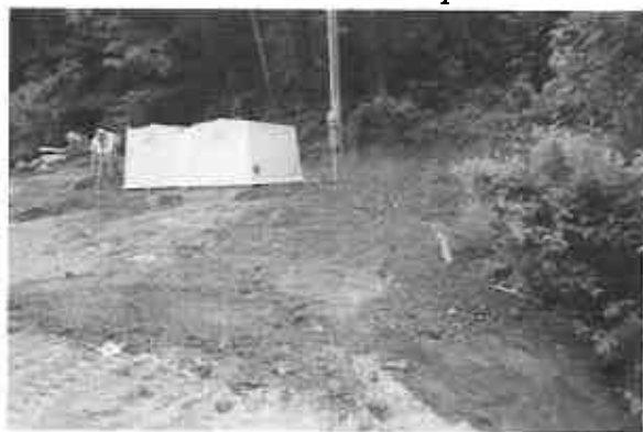
New booster station during construction.
