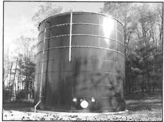
402,000-Gallon Water Storage Tank
