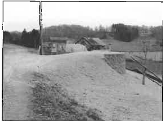
50 GPM Booster Station
