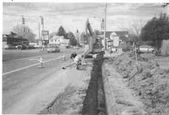
Replacement of water line along US Route 60.
