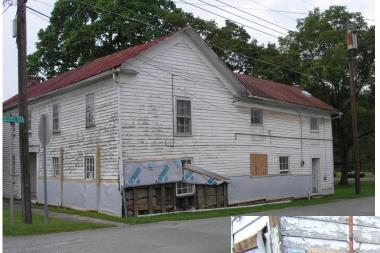
The original portion of this structure was constructed as a log cabin in the 1770's. This project included foundation stabilization and log wall and floor framing repairs.
