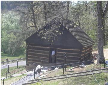
The uphill wall was exhibiting damage due to the condition of the beam at the top of the wall, allowing the wall to push out from thrust on the deteriorated beam.
