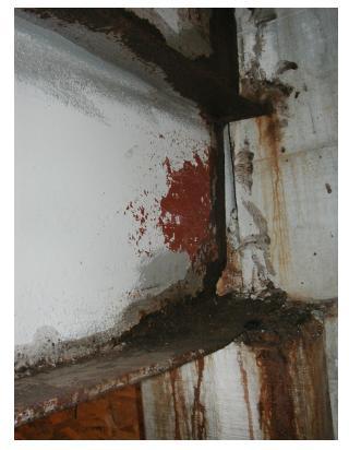
A steel pipe column was added below the bearing end of this beam due to the severe deterioration at the end of the beam.
