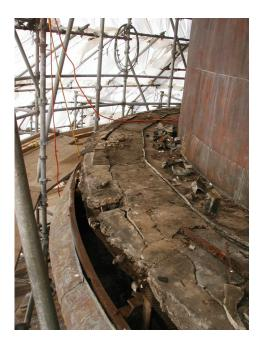
Concrete at the railing level was hidden from view and repaired once the sheet metals was removed and the deterioration was found.
