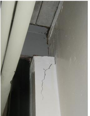
The pool deck is supported by this structure, thus the severe deterioration due to leaking joints in the deck. Once the decking is repaired, a new coating system must be installed to prevent chemically treated water from deteriorating the structural members.
