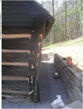
The structure was originally constructed of local poplar trees and clay chinking. A replacement log was hand hewn to the required size for the beam on the uphill side. Epoxy repairs were made to the beam on the downhill side. A team of horses brought the log to the site.
