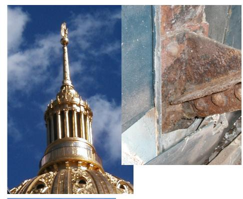
The structural steel in the lantern level shows evidence of deterioration. Project included probing to determine extent of deterioration and preparation of plans and specifications for repairs.
