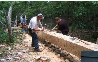
This log structure was constructed in the 1860's, having begun prior to the Civil War and completed afterward. The years had taken a toll on the main logs/beams at the top of the walls supporting the roof structure.
