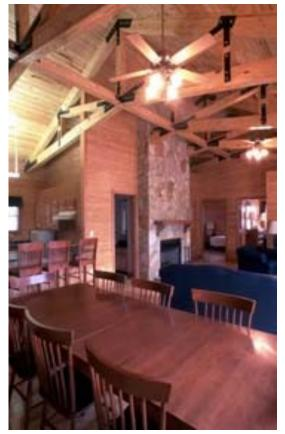
The project included design of new cabins with exposed glulam scissors roof trusses.
