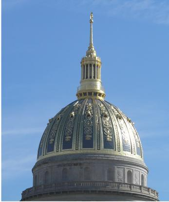
Completed dome restoration shows the original sheet metal detail on the previous lead coated copper sheet metal. The lead coating was compromised over the years. As a result, a coating system had to be applied to protect the copper sheet metal.
