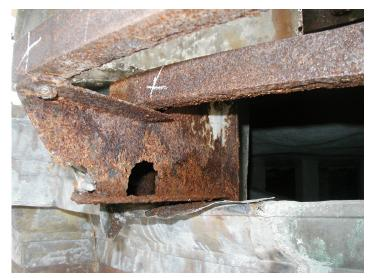
Deterioration of steel supporting sheet metal exhibited such deterioration that portions of the steel have disintegrated.
