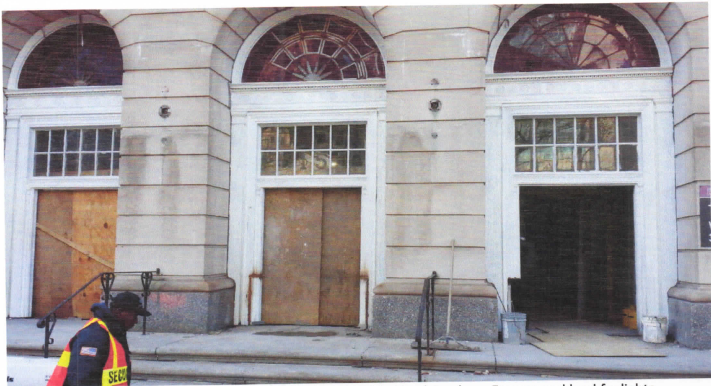
Jams all cut away over 2' high, repaired in shop, and welded back in place. Frames and lead fanlights stripped and frames repainted.
