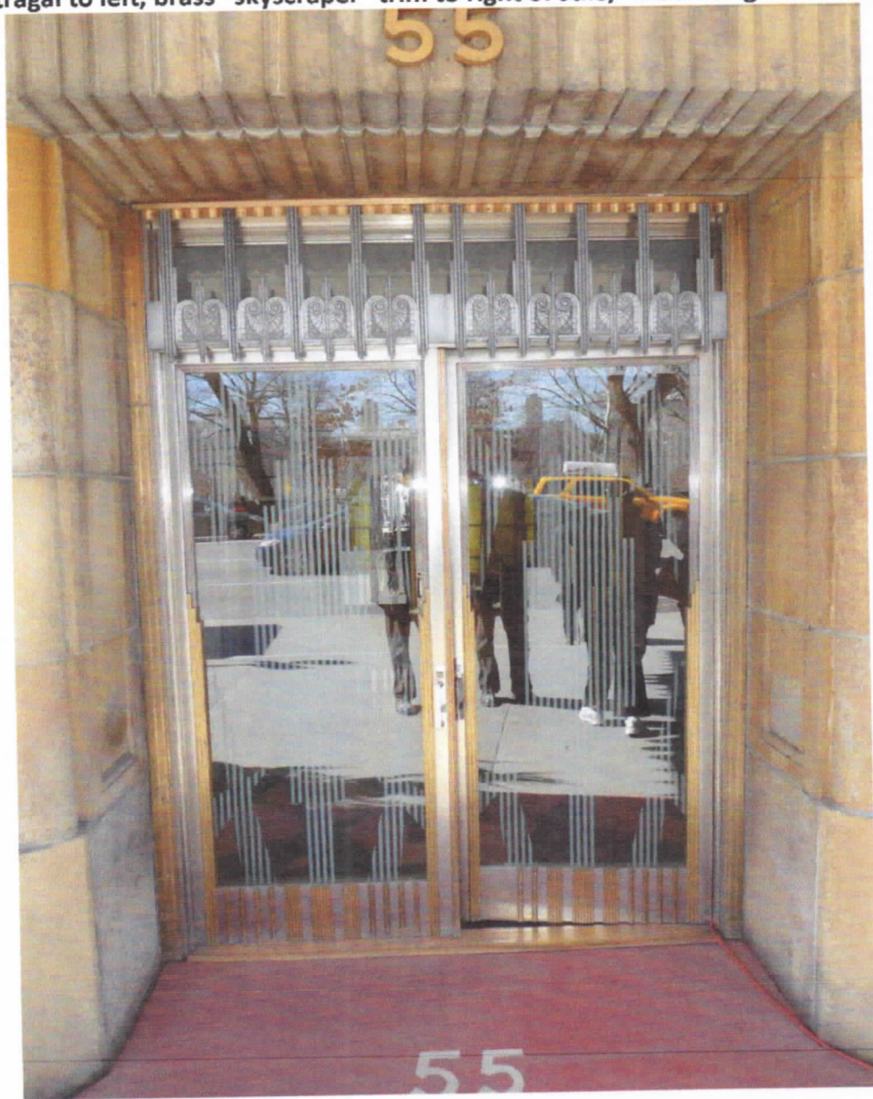
New Door astragal to left, brass "skyscraper" trim to right of stile/ Machining trim moldings
