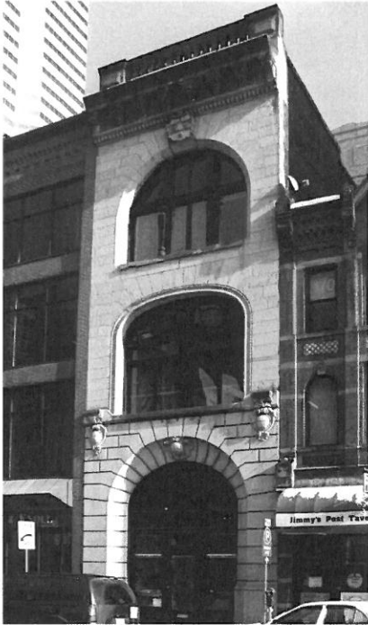
PWWG's office in a former City firehouse in downtown Pittsburgh
