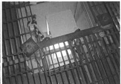
ZMM completed the Great Hall Wiring System located at the Cultural Center on WV State Capitol Complex. The existing wiring and conduit system was approximately thirty-five years old and in need of drastic improvements. The existing conditions that were observed included the conduit and outlet boxes were mounted on the underside of the existing grating above the ceiling, the dimming circuits shared a common neutral, bad fixture connections and cables.
