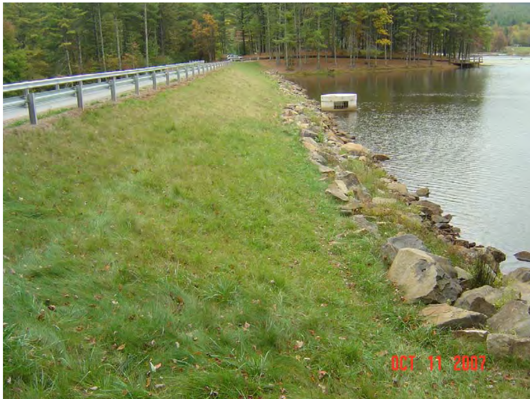
MONCOVE DAM MODIFICATION, MONROE CO., WV
