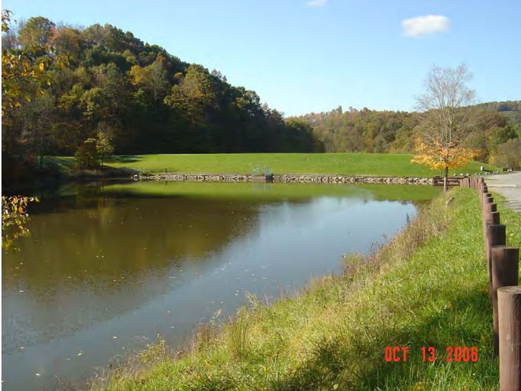
JIMMY LEWIS DAM MODIFICATION, MERCER CO., WV
