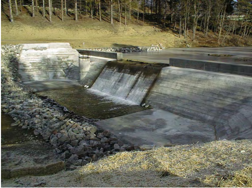
THOMAS DAM MODIFICATION, THOMAS, WV
