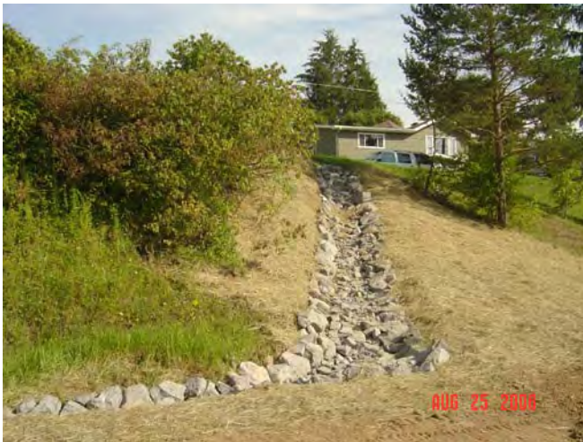
Erosion Repair – Rip Rap Armored Ditch
