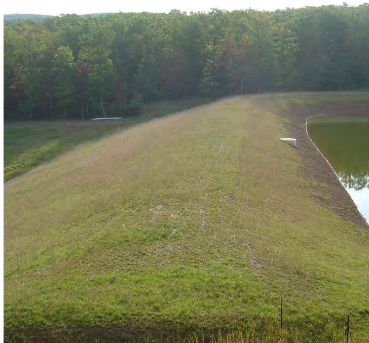
WILSON DAM MODIFICATION, HAMPSHIRE CO., WV
