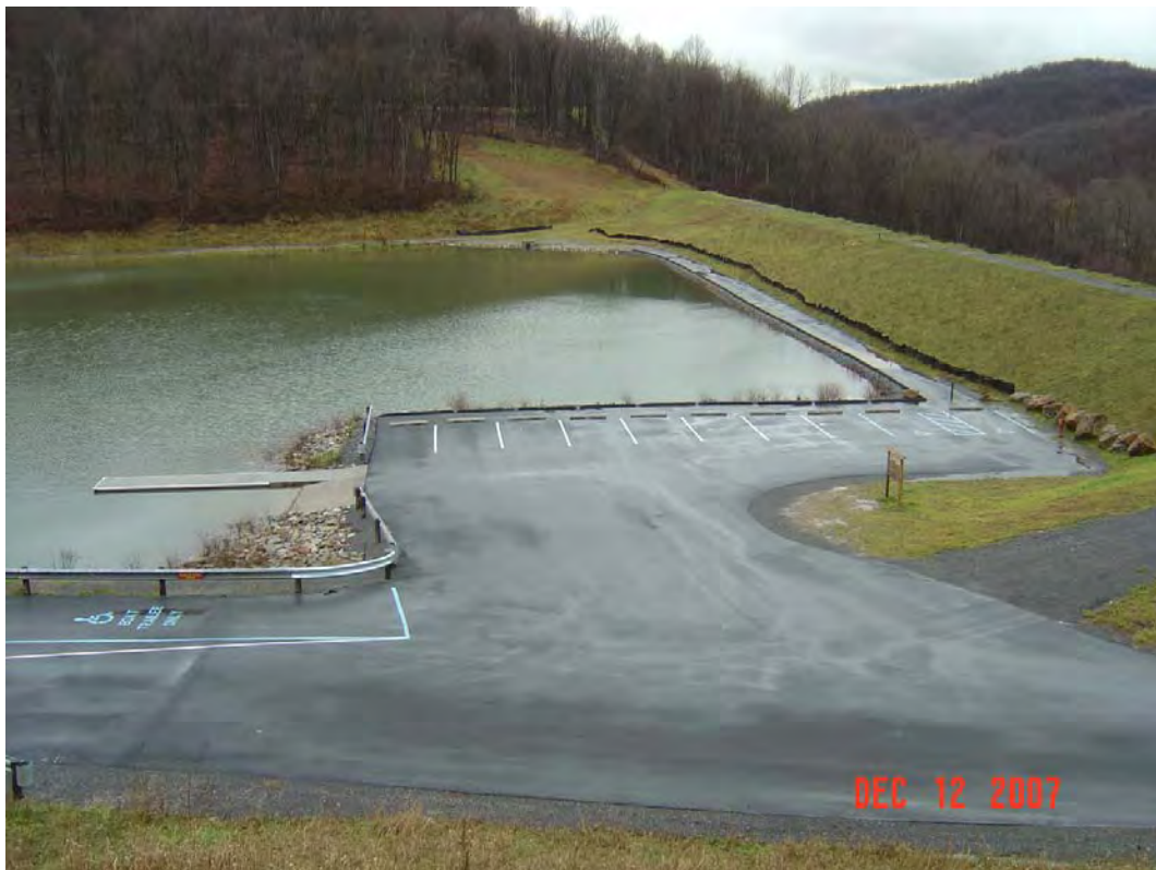
BAILEY DAM MODIFICATION, MONONGALIA CO., WV
