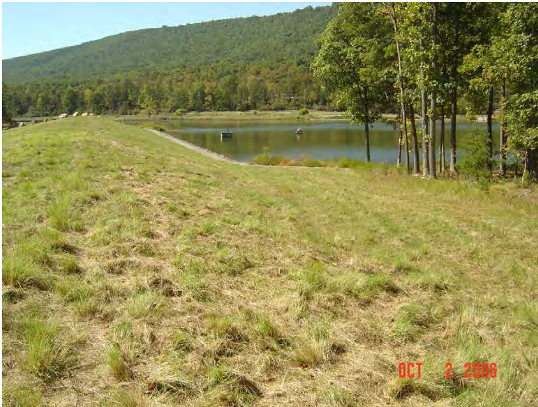
WARDEN LAKE DAM MODIFICATION, HARDY CO., WV
