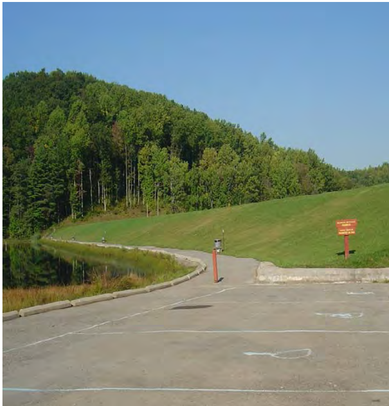
TETER CREEK DAM MODIFICATION, BARBOUR CO., WV
