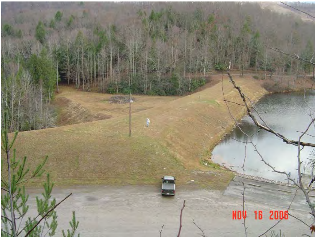
PLUM ORCHARD DAM MODIFICATION, FAYETTE CO., WV
