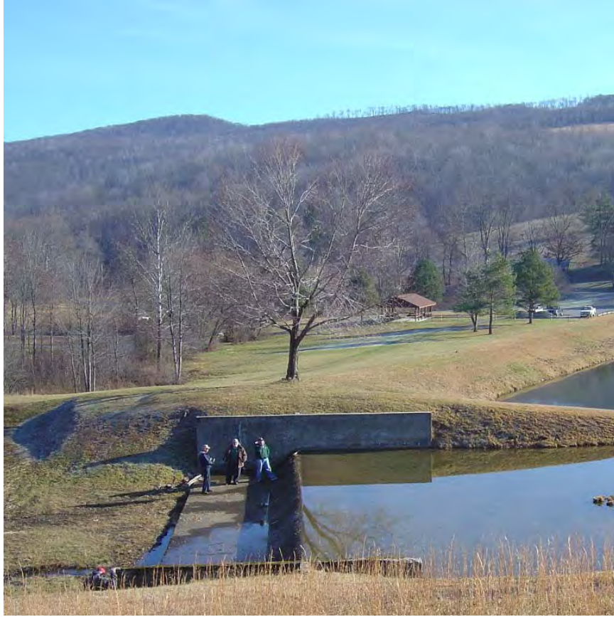
BELINGTON DAM MODIFICATION, BELINGTON, WV
