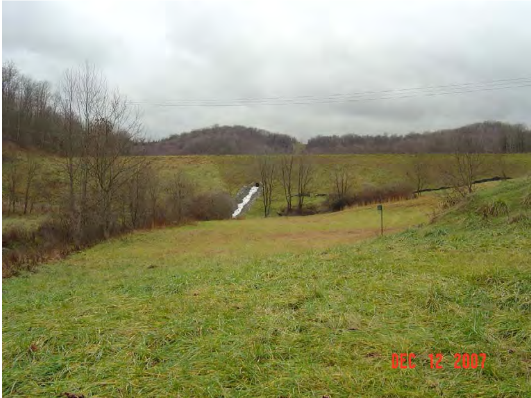
LEMLEY DAM MODIFICATION, MONONGALIA CO., WV
