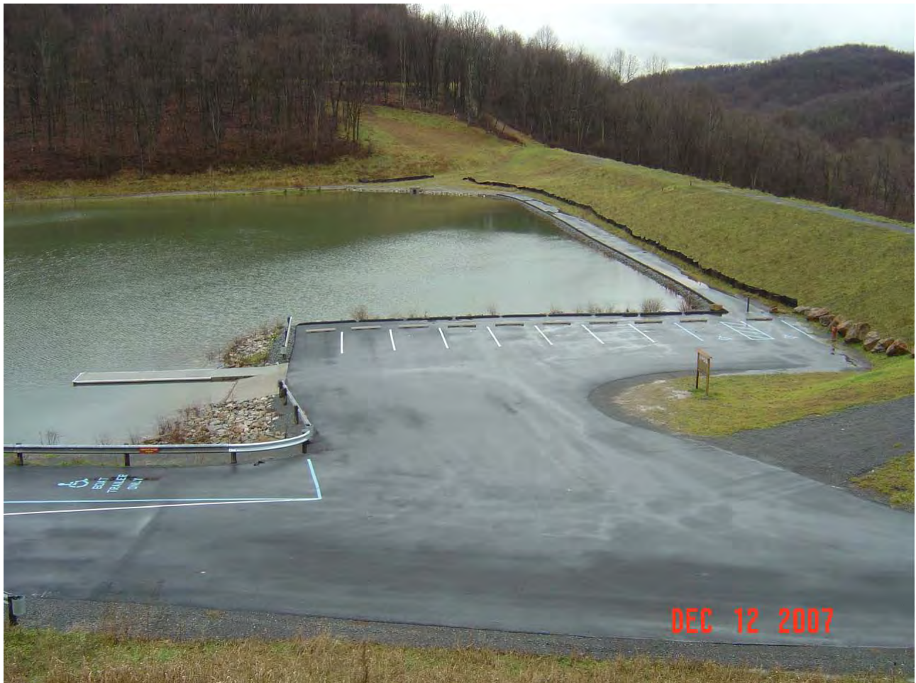
MASON DAM MODIFICATION, PARKING, BOAT LAUNCH, COURTESY DOCK MONONGALIA CO., WV
