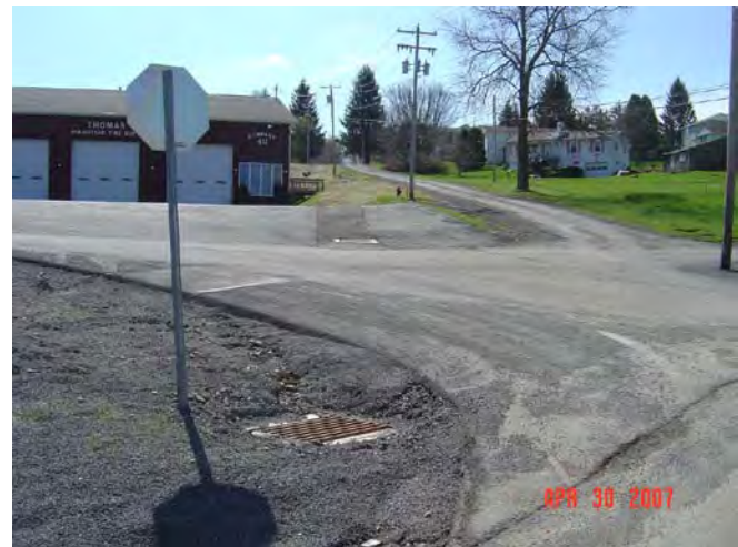
New Storm Drains and Catch Basins
