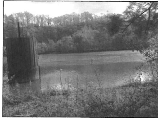
Monongahela River – Project Site Before Construction
