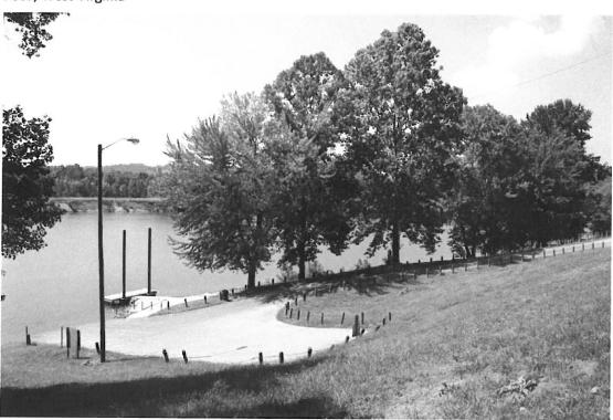
The project consisted of a 30 space combined boat trailer and automobile parking lot, including handicapped parking; an ADA accessible ramp and railing; a stationary pile driven fishing pier; and all required permitting.
