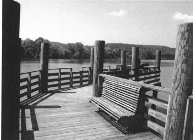
The project consisted of a 30-space combined boat trailer and automobile parking lot, including handicapped parking; an ADA accessible ramp and railing; a stationary pile-driven fishing pier; and all required permitting.
