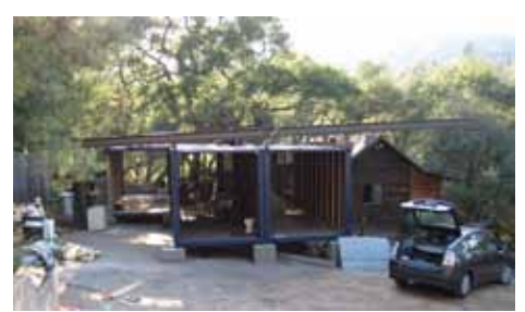
Container House — Topanga Canyon, California Modern POD design using retrofitted shipping containers. Dramatic, long-span cantilever roof in near-fault seismic zone.
