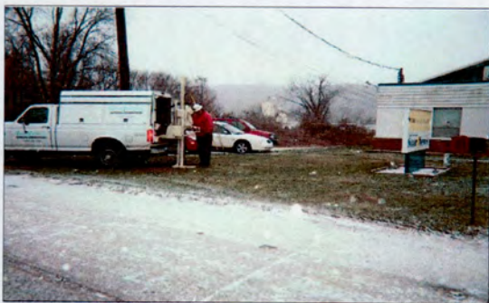
Soil Boring During Limited Phase II ESA
