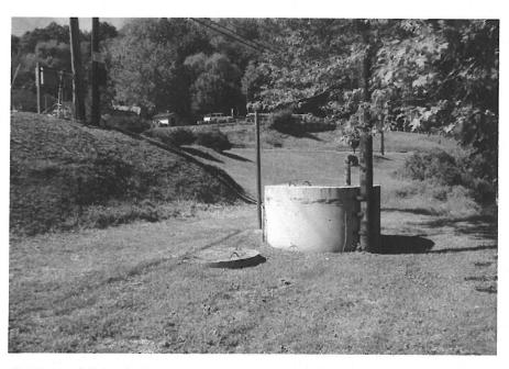
Portions of the existing sanitary sewer collection system in the Town of Wayne are Combined Sewers, which convey both sanitary sewage and storm water. During the periods of heavy rainfall, the storm water exceeds the capacity of the combined sewers and overflows into Twelve-pole Creek.
