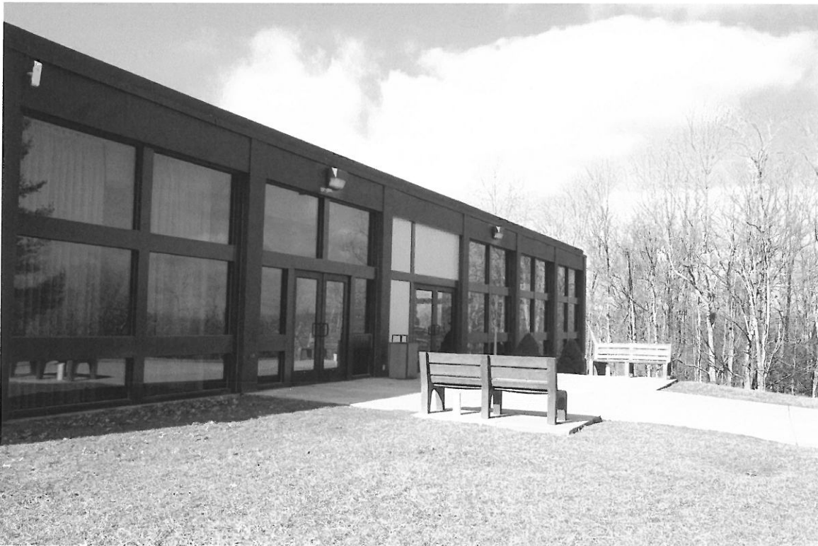
Pipestem Conference Center Addition
