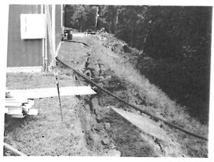
Potesta & Associates, Inc. (POTESTA) was retained by Columbia Natural Gas (Columbia) to evaluate and design remedial measures for a landslide at Columbia's Clendenin Compressor Station. The landslide was located adjacent to the office and maintenance building at the facility and threatened to damage the structure.
